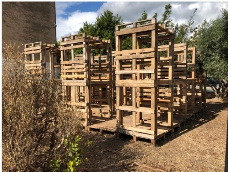
The edible shelter under construction
